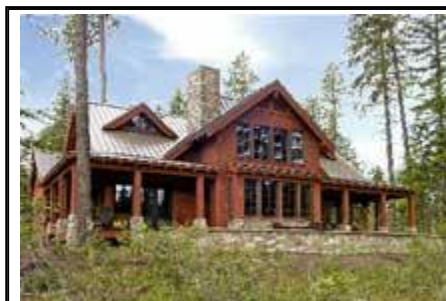
CMI Homes' Built Green showcase home is located in Suncadia, a resort community about 15 minutes east of Seattle. The natural landscape outside of the building envelope was left untouched.
